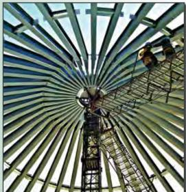
Sukup offers commercial roofs with 15,000, 30,000, 50,000 or 100,000 lb. peak load ratings. Roof ratings are pounds evenly distributed on peak ring as pure vertical load with uniformly distrubted roof snow load calculated from 40 psf ground snow zone or 105 mph wind zone as defined by ASCE7-10 Code.
