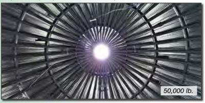
The strength of the 30,000 lb. Sukup roof comes from double C-shaped channels forming I-beam rafters with C-shaped purlins. Rafters and purlins are manufactured from 70,000 psi tensile strength galvanized steel. The rafters in the 156' bin are constructed with 65,000 psi tensile strength I-beams.
