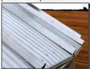
the ribs two different widths for a better overlap and fit. The inner or lower rib is slightly smaller than the upper, allowing the sheets to nest properly.
